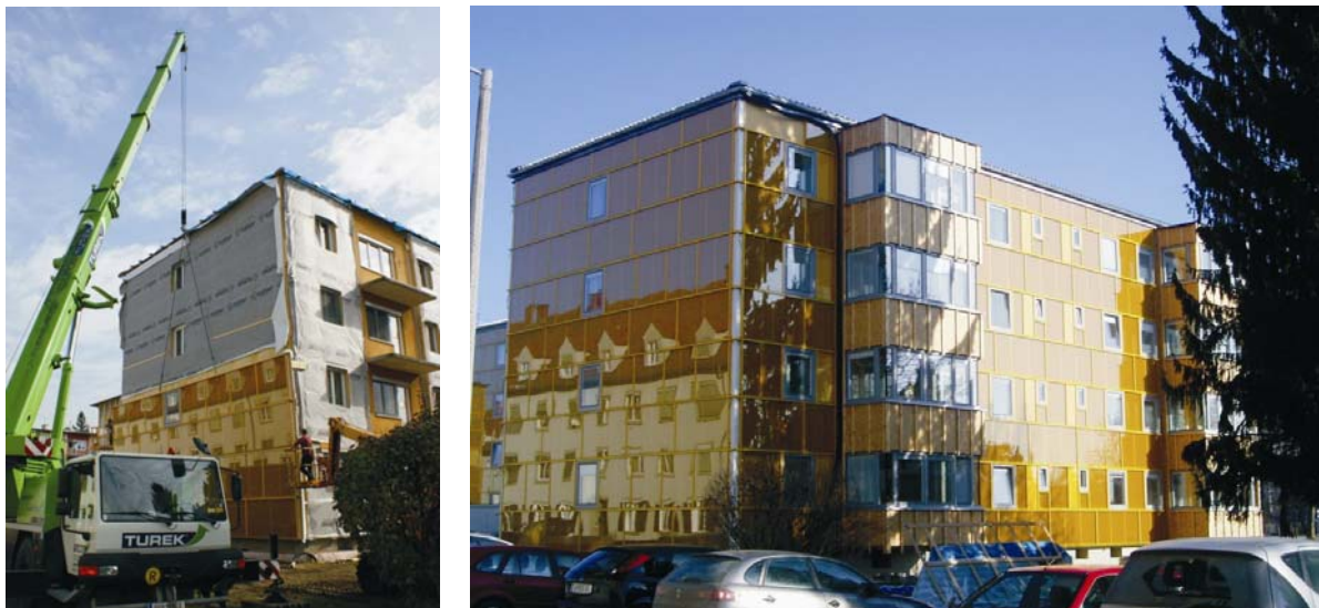
Figure 4.9 and 4.10 Pictures of the construction work (left side) – the pre-fabricated modules are brought by a truck and trailer on-site. Afterwards they are lifted by a truck-mounted crane to the buildings façade. The picture on the right side shows the new envelope – with the integrated balconies (to be used as additional living space)
