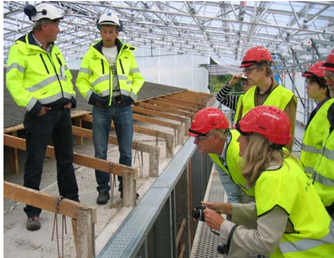
Figure 3.7 and 3.8 Protecting a building site and stored materials often pays back as improved work efficiency even though the main purpose is to avoid moist/damp construction parts and mould growth.
