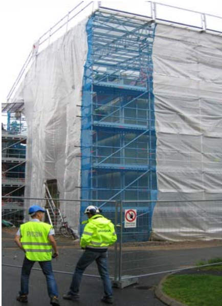
Figure 3.7 and 3.8 Protecting a building site and stored materials often pays back as improved work efficiency even though the main purpose is to avoid moist/damp construction parts and mould growth.
