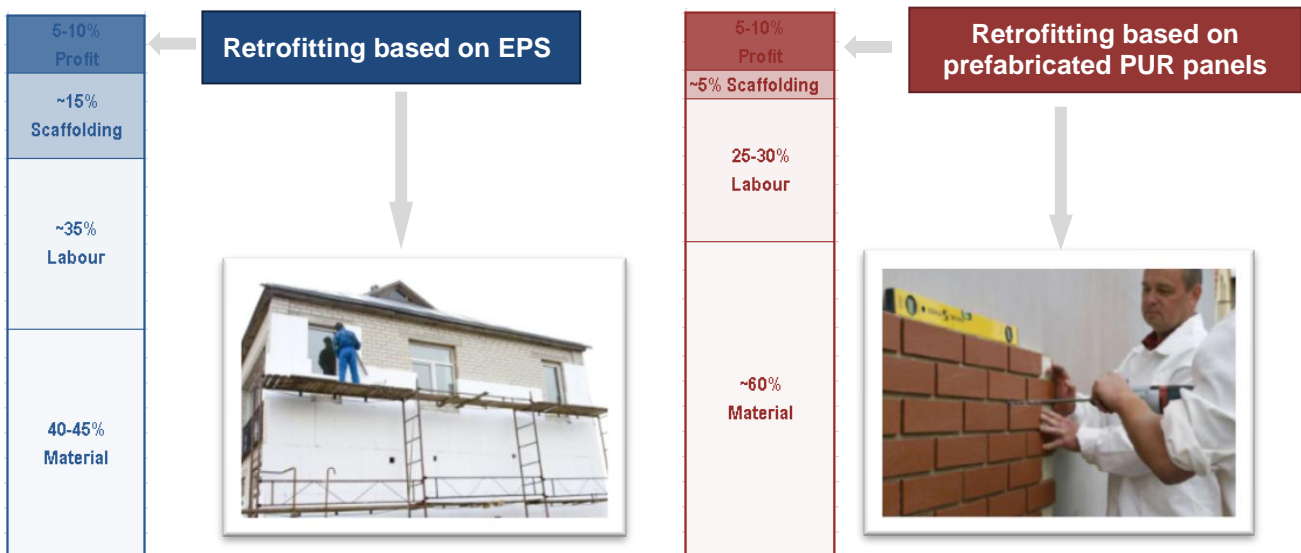
Figure 31 - Cost structure of two retrofitting solutions based on EPS and prefabricated PUR panels. Based on internal data of PRE Fasada
