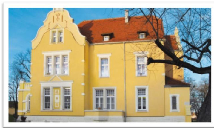
Figure 21 - Kindergarten retrofitted with the use of phenolic foam panels in Dzierżoniów in Poland
