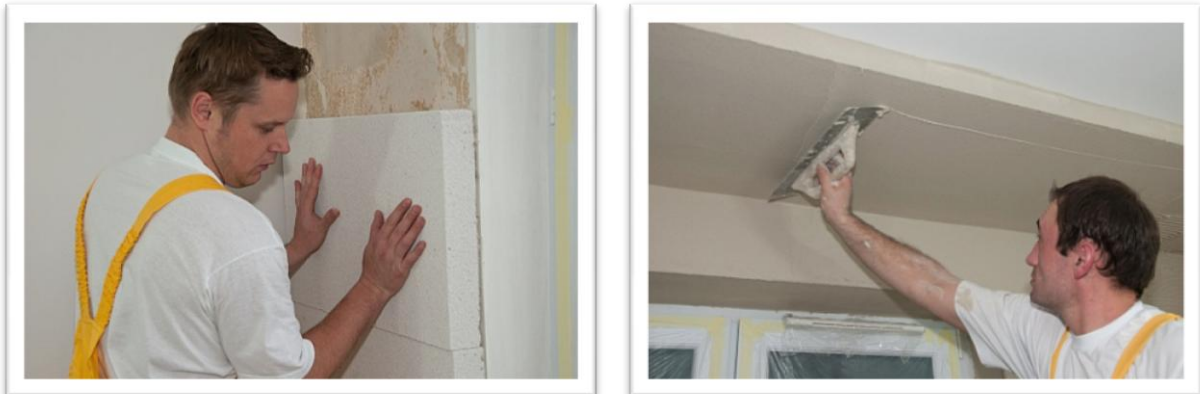
Figure 24 - Internal insulation with the use of Aerated Autoclaved Concrete blocks – Ytong
