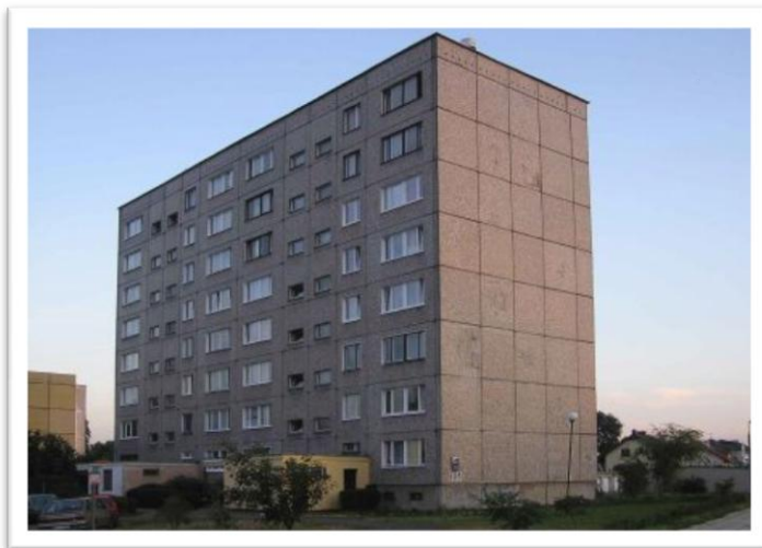
Figure 11 - Example of a building constructed in prefabricated panel technology – not retrofitted in Poland
