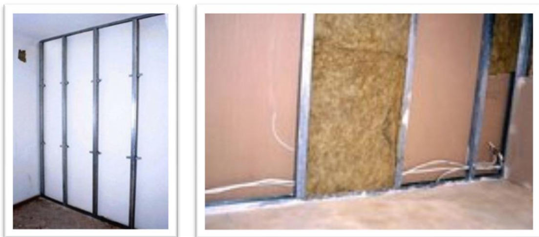
Figure 23 - Internal insulation with the use of mineral wool
