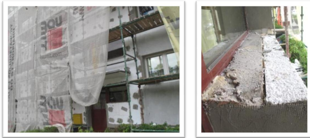
Figure 15 - Building during retrofitting works with EPS system in Poland
