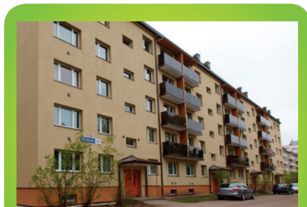
Refurbishment work using KredEx fund Photo credit: Mirja Adler, KredEx
