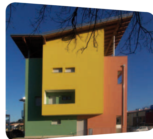
Fig. 16 – IRH-Med pilot in Pesaro (I): sizing thermal inertia of external walls in accordance of solar orientation.
