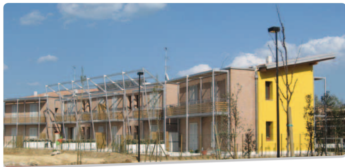
Fig. 17 – IRH–Med pilot in Pesaro (I): using external desolidarized Southern balconies as shading devices and support for solar thermal and PV panels.
