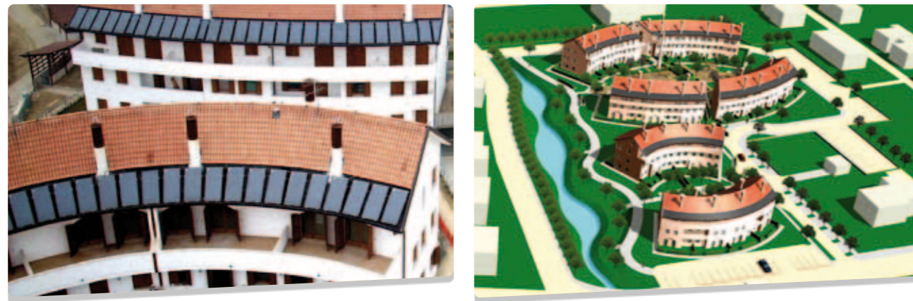
Fig. 20 – Social Housing neighbourhood in Preganziol (I): harvesting rainwater and at reusing treated grey water with sustainable sanitation. Source: www.she.coop – European VFP demonstration project.
