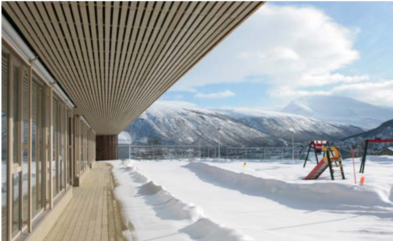
Figure 1; Kvamsstykket passive house kindergarden, Tromsø, Norway. Architects and landscape; Arkitekturverkstedet/ Asplan Viak, Oslo and Tromsø. Photos: Asplan Viak
