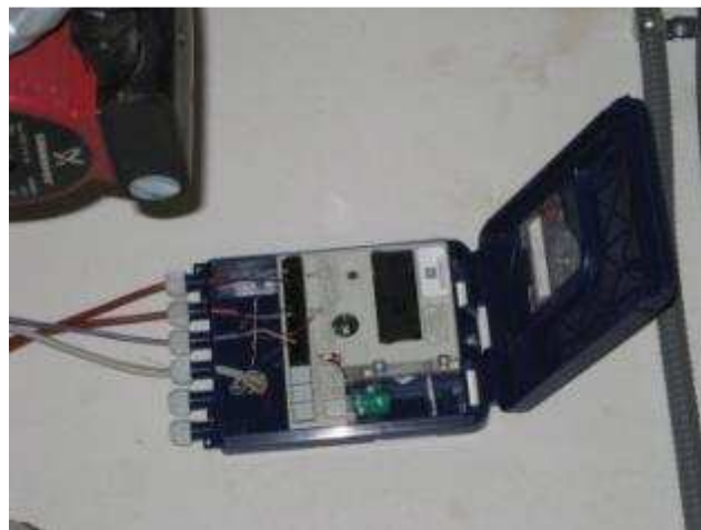
Figure 14: Installation of solar thermal generation monitoring system
