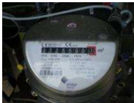
Figure 2: Counter at the Genoa pilot that does not support telemetry – photo from the technical visit
