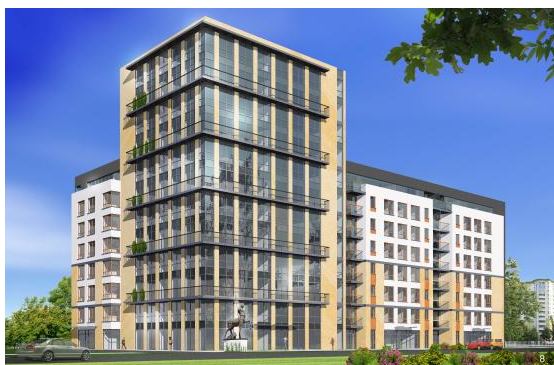
Multi-family residential building in Brussels, Belgium where one of the TRAINREBUILD training events took place
