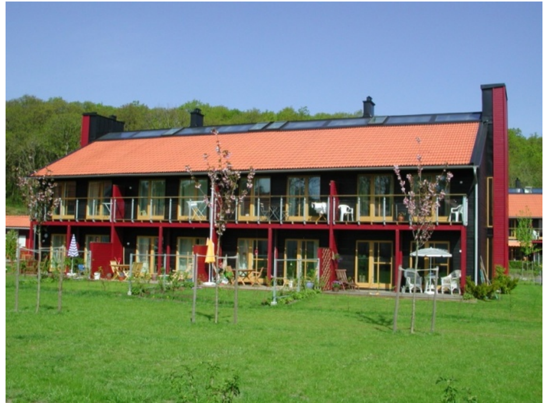
Passivehouse Lindåsen. Photo Maria Wall
