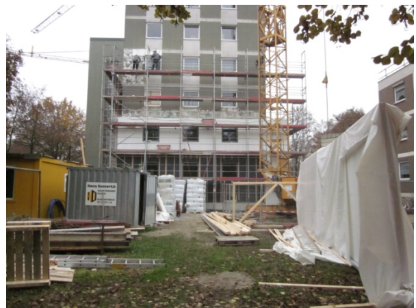
Figure 14 - Protection during site storage
