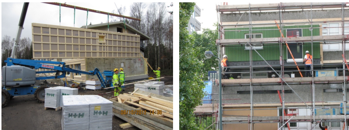
Figure 8 - Oulu: mounting with lift platform. London: crane mounting with scaffold
