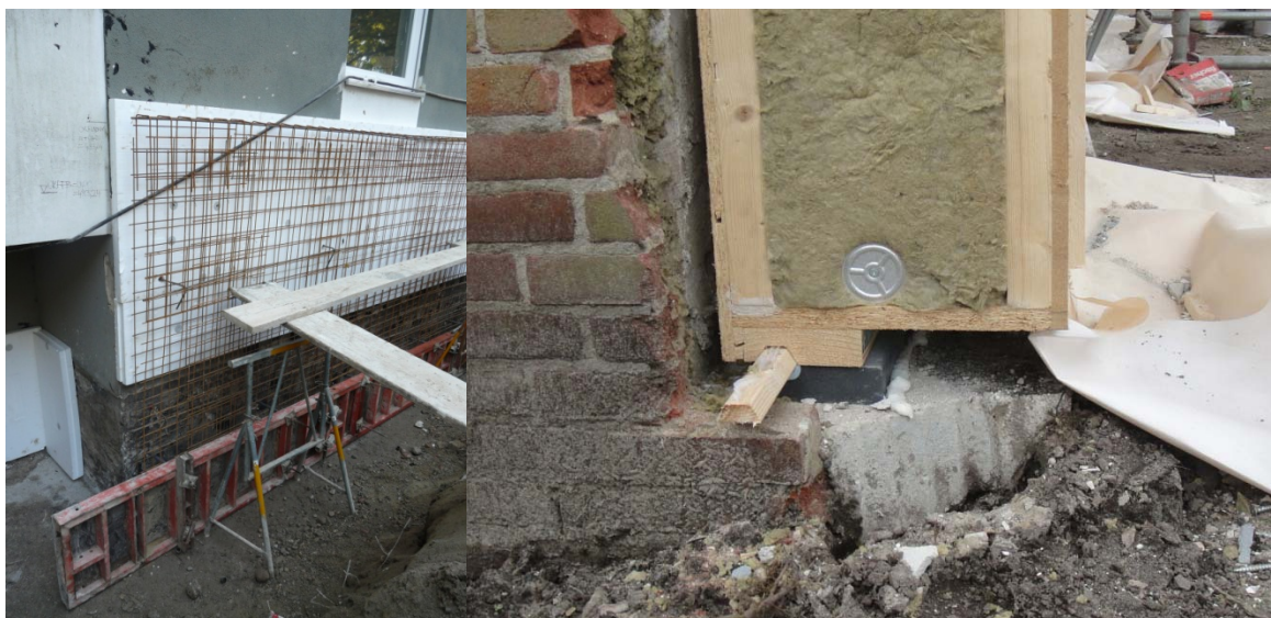
Figure 16 - Additional foundation, Augsburg and Roosendaal
