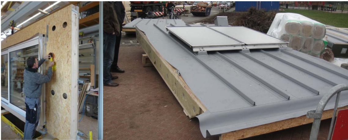
Figure 4 - Element production (Gumpp & Maier, D-Binswangen). Roof element Roosendaal
