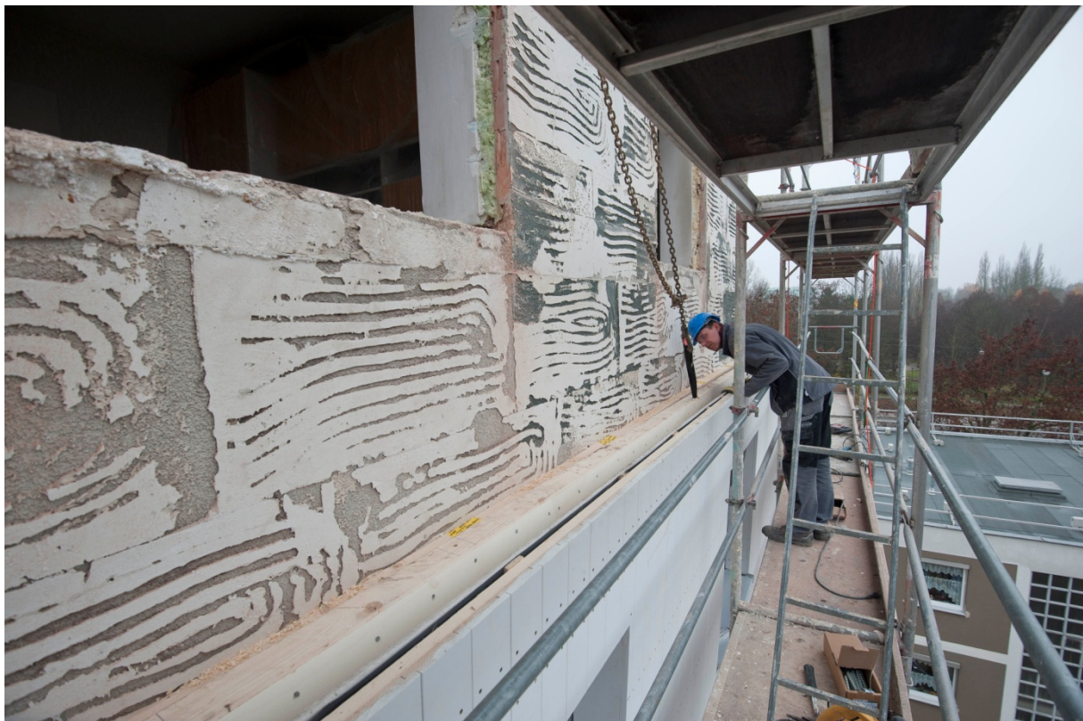
Figure 9 - Facade assembly, window removed to the outside
