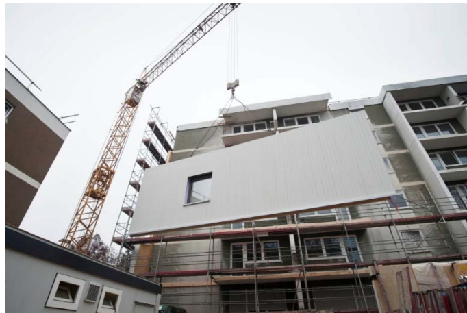
Figure 6 - Augsburg: elements are lifted by tower crane
