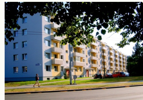
Renovated buildings in Estonia managed by apartment associations (divided ownership)
