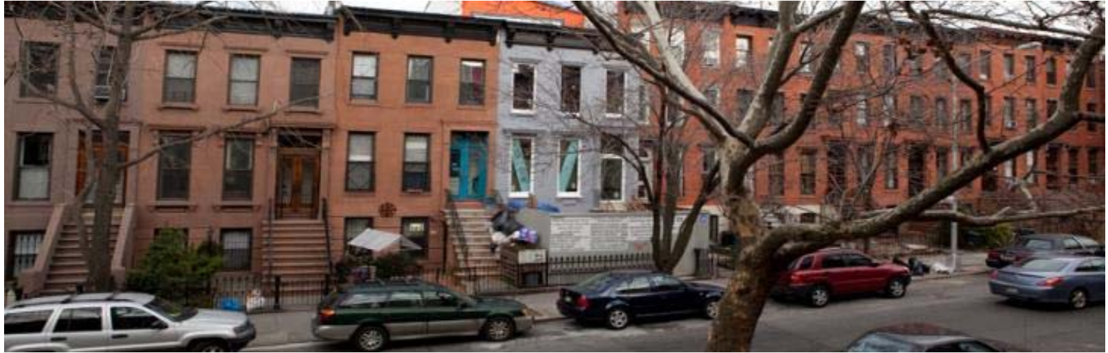
Architect: Julie Torres Moskovitz the 'Tighthouse' project: 23 Park Place, Brooklyn, NYC
