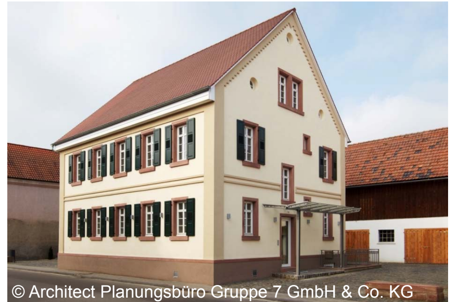
After refurbishment: 20 kWh/(m 2 a)
