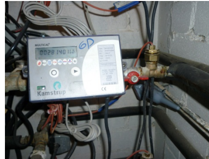
ISA NetMeter connected to individual heating counter
