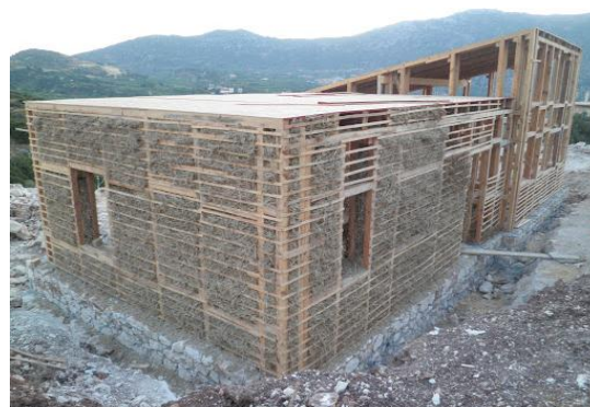
Straw/clay walls construction, residence in Archanes (Crete), Greece
