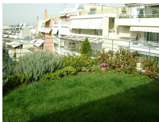
Green roof (extensive) on residential building, Athens, Greece
