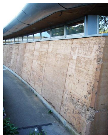
Rammed earth walls, EDEN Project, Cornwall, UK
